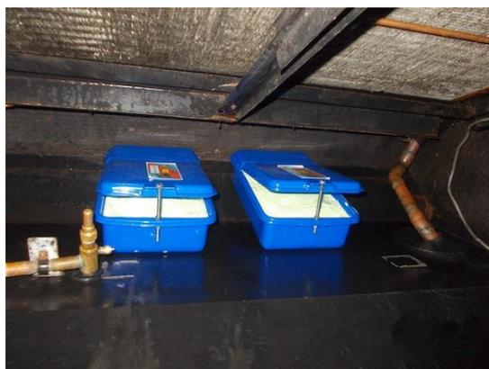
For best results the opening of the box should toward the airflow. See diagram.
